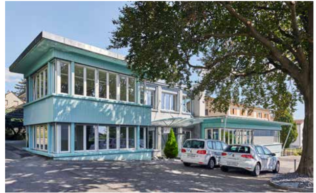
Assembly workshop Grenchen / warehouse
